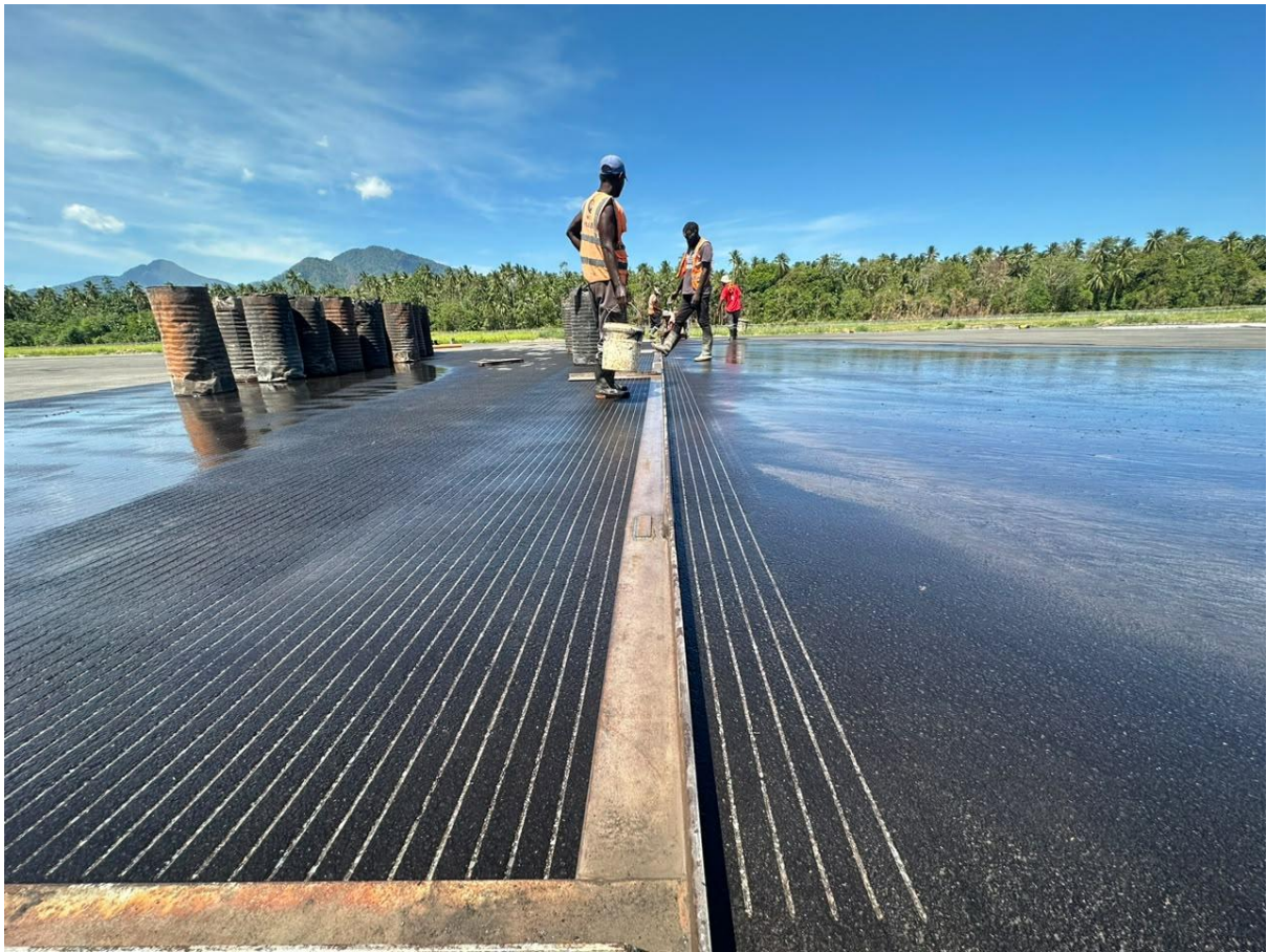
Caption 3: Grooving works in progress under MOWP Stage 10.
