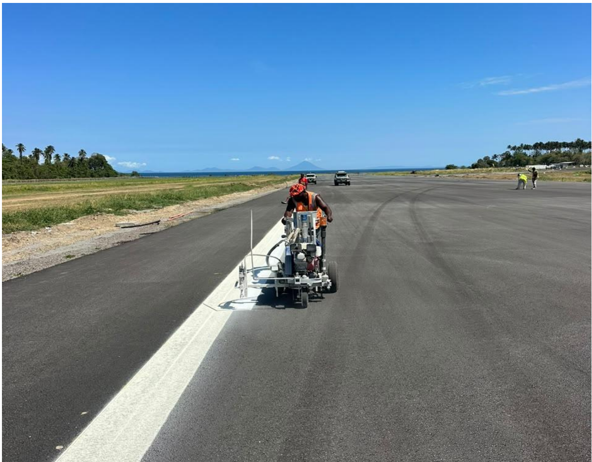
Caption 4: Line marking in progress under MOWP Stage 10.
