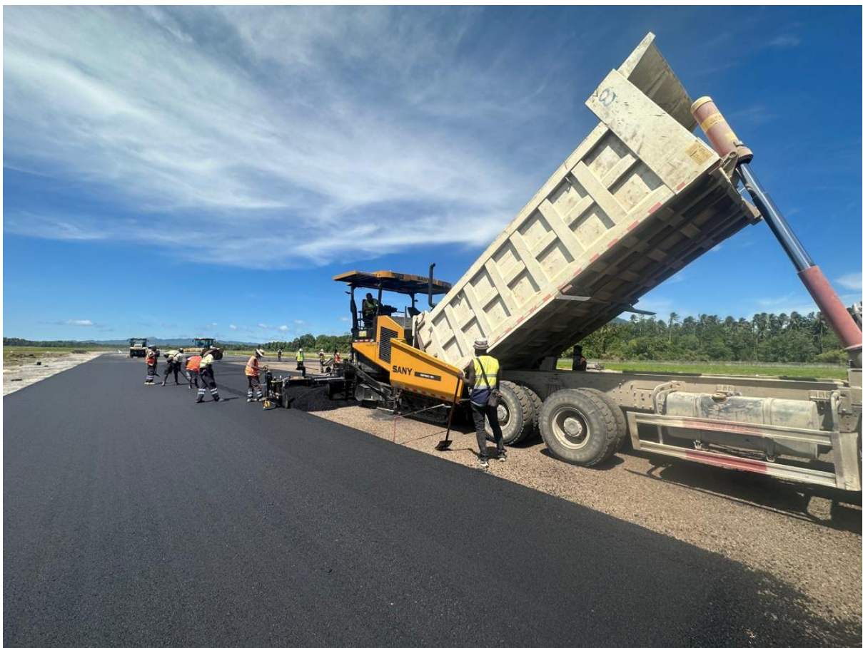
Caption 2: Asphaltting works in progress under MOWP Stage 10 at Hoskins Airport.
