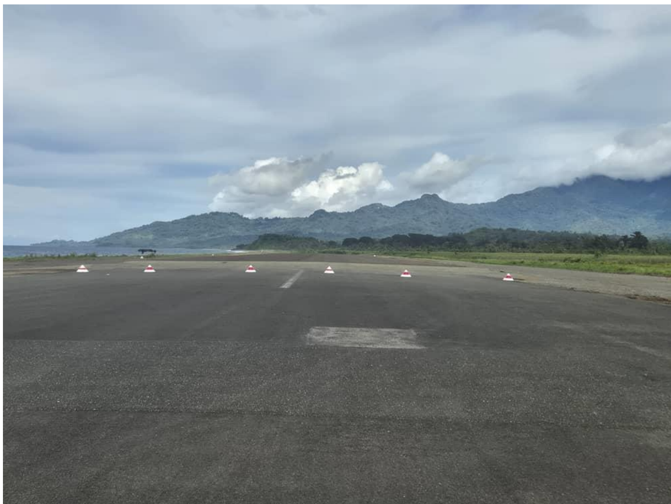
Caption 1: Construction works on the runway at Kieta Airport in progress.
