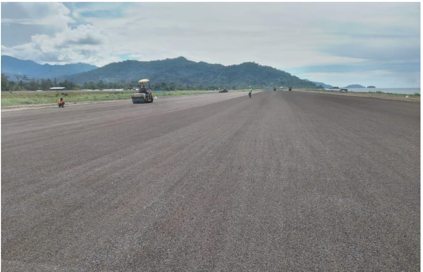
Caption 2: Runway Surfacing/Chipseal in progress at Kieta Airport.
